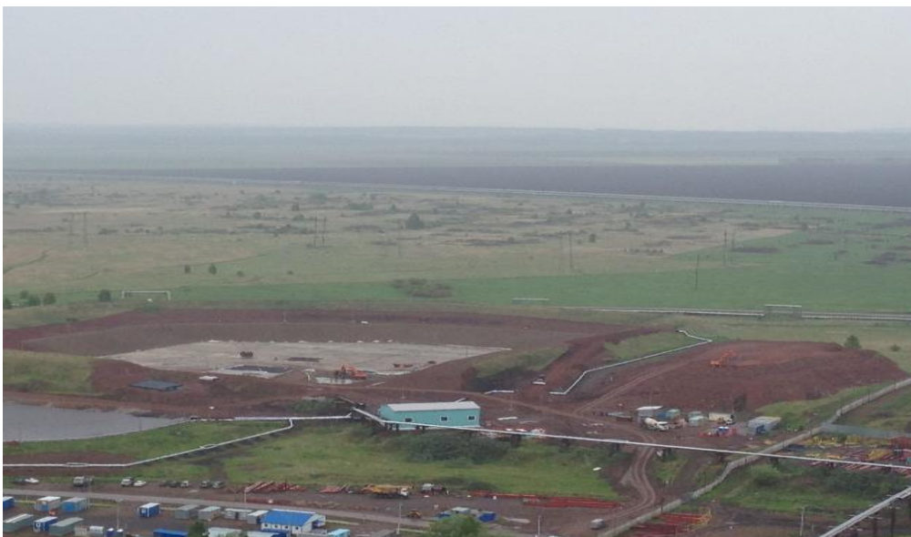
Construction of the dry ash and slag removal system
