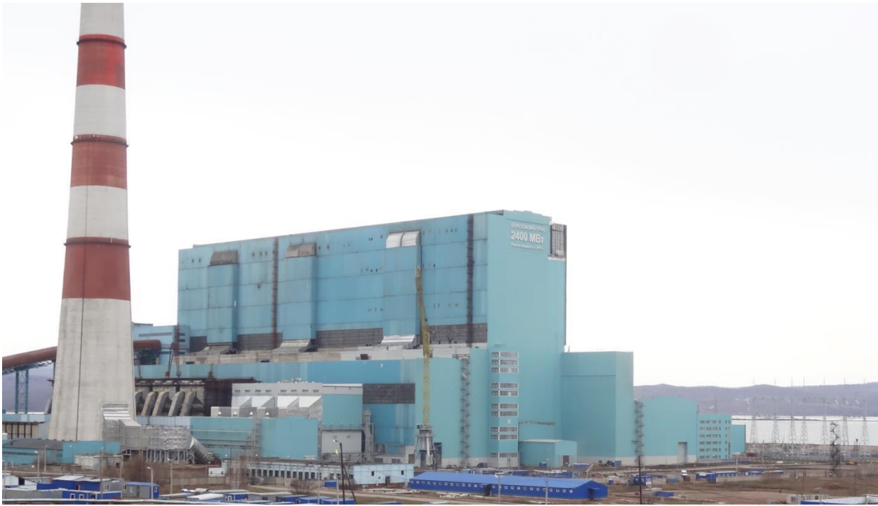
Power unit No. 3 of Berezovskaya GRES
