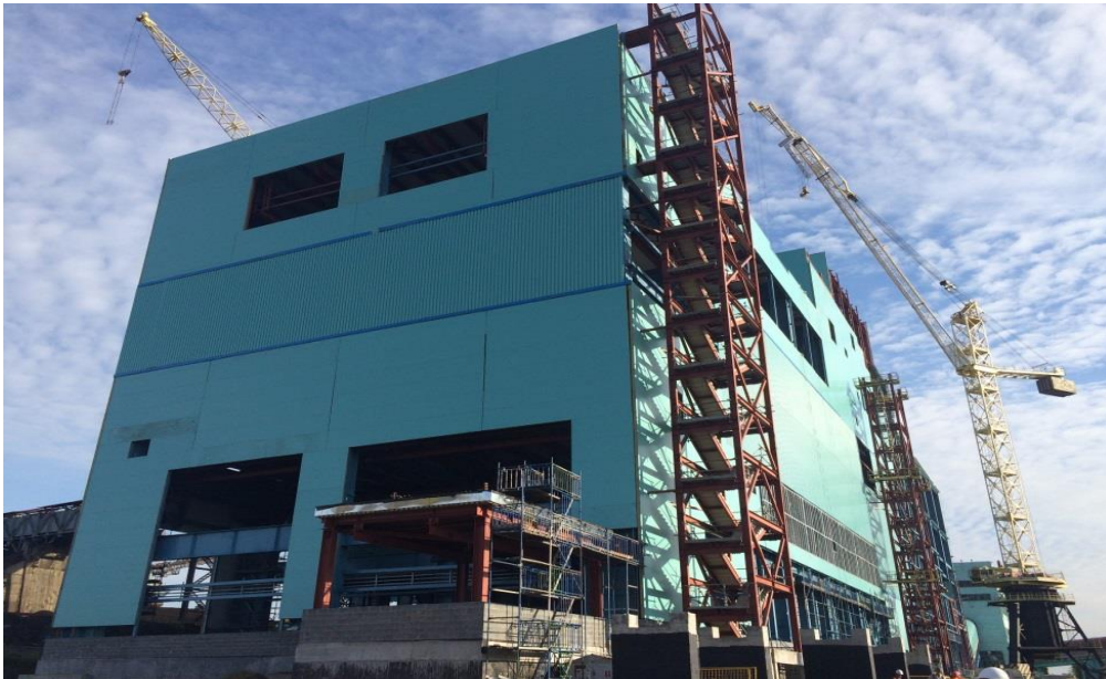
Fuel receiving station
